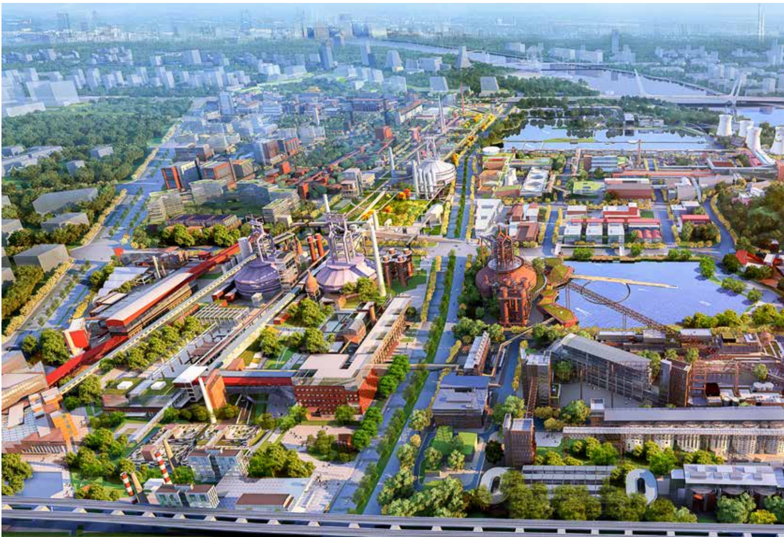
▼ 新首钢高端综合产业服务区 An aerial view of Shougang Park
